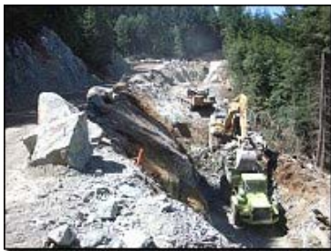
Pipeline Ditch Construction
