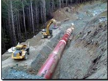
Pipeline Backfill
