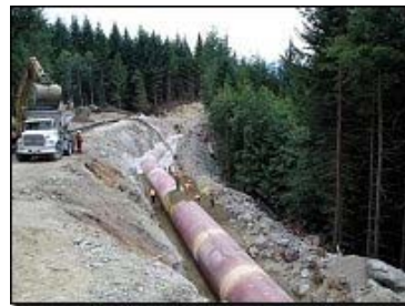
Pipeline Ditch Construction
