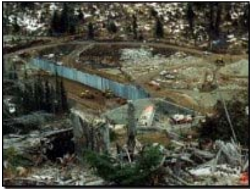
Pingston Dam Construction
