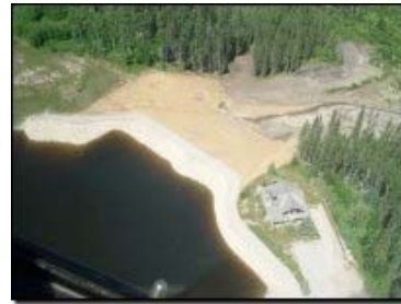
Priddis Dam Construction
