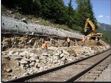
Soil Anchor Wall Construction
