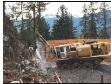
Site Preparation Coast Hillcrest Hotel
