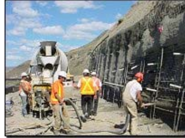
Soil Anchor Wall Construction
