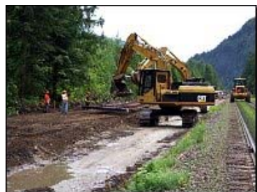
Railway Siding Extension
