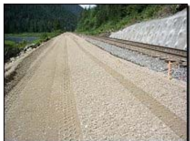
Railway Siding Extension
