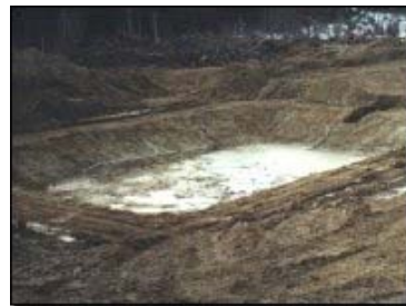
Settling Pond Construction
