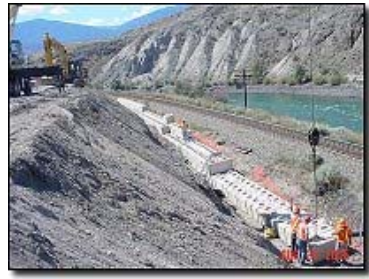
Lock Block Wall Construction
