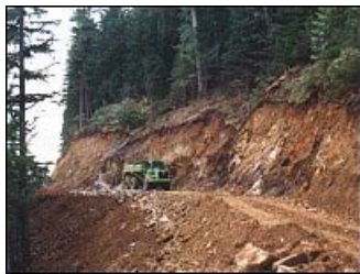
Forestry Road Construction
