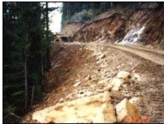
Forestry Road Construction
